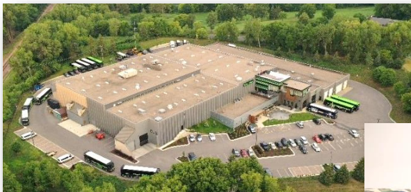
Existing SWT Eden Prairie Bus Garage Roof
