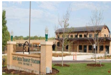
East Creek Station
